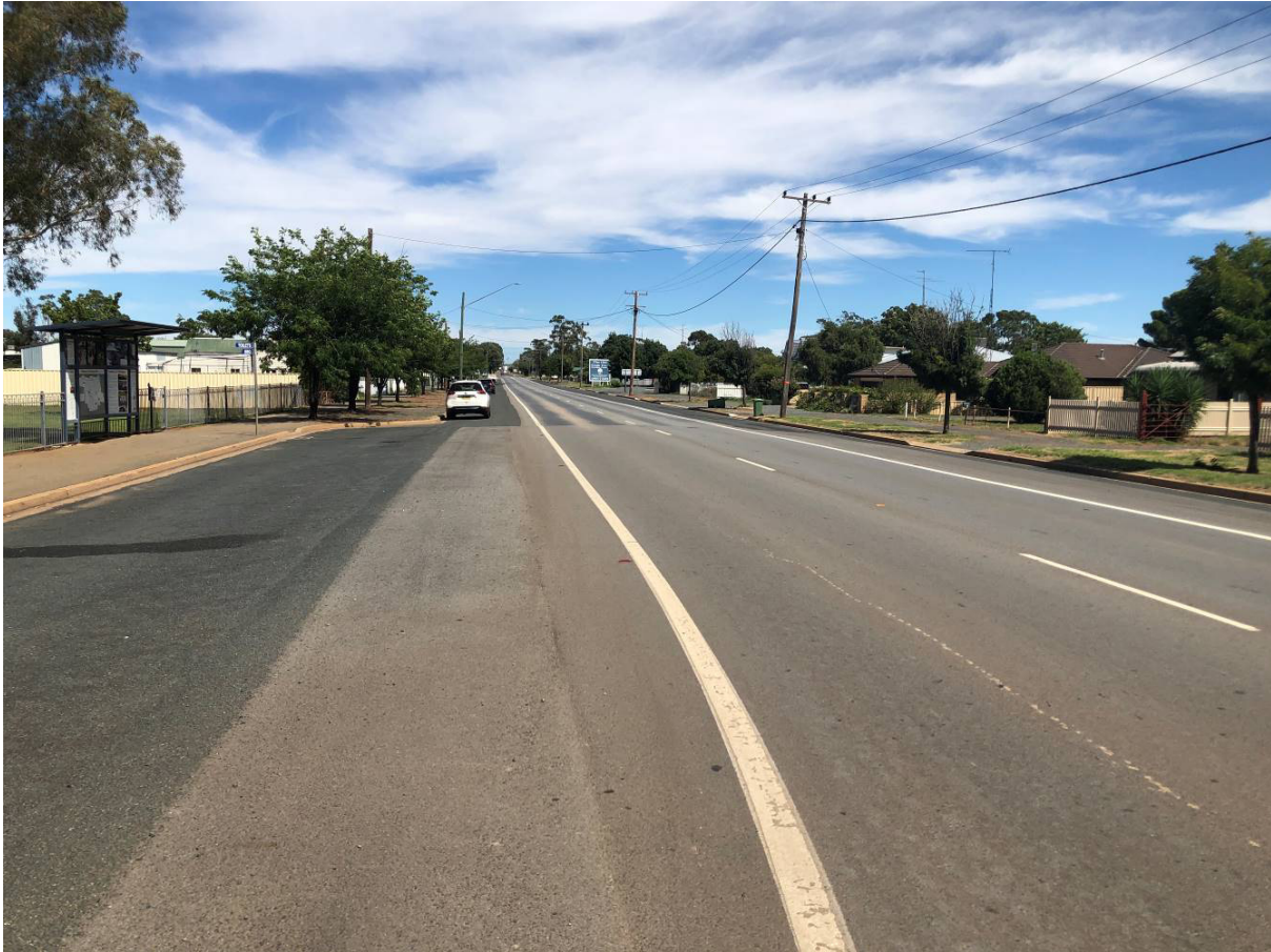
Photograph 3 – Newell Highway through Wyalong
